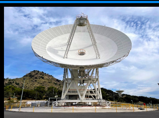
Deep Space Station 53 is a new waveguide antenna that went online in February 2022 at NASA's Deep Space Network's ground station in Madrid
