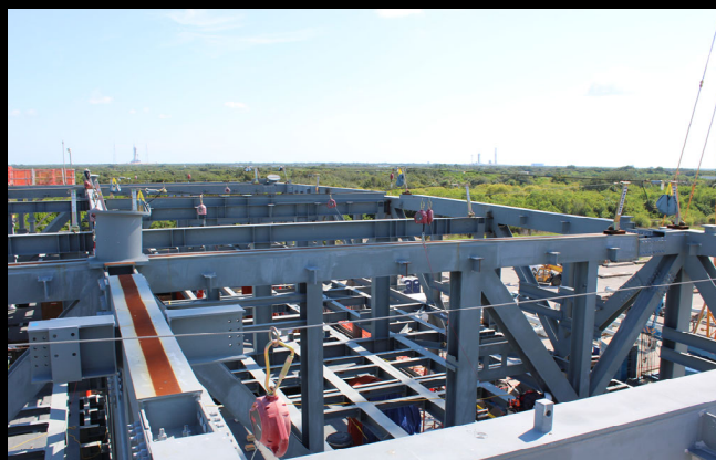
Progress on the ML2 base build-out as seen from above as of August 20, 2024
