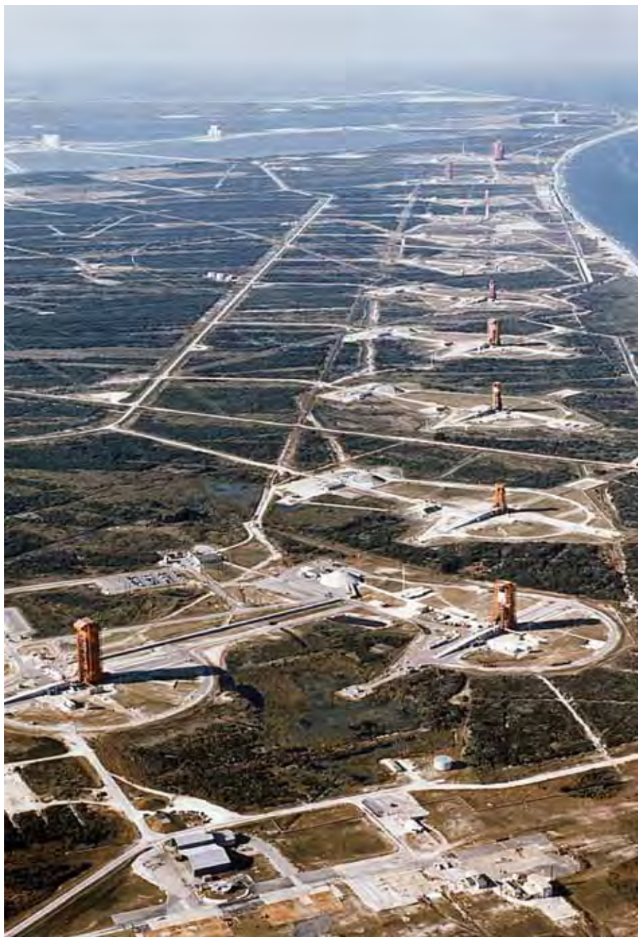
Figure 3: Spaceports were also essential infrastructure for the Age of Space. This aerial view of Missile Row, Cape Canaveral Air Force Station, was taken in November 1964. The view is looking north, with the VAB under construction in the upper left-hand corner. NASA Image 64PC-0082
