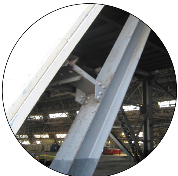
Figure 3-4: Wind Girt @ 7'-6" O.C.
