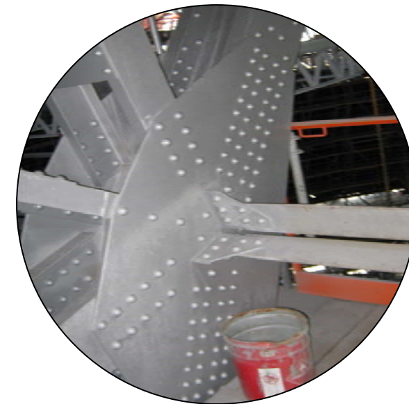
Figure 3-11: Bottom Chord Connection
