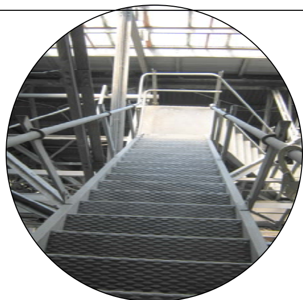
Figure 3-2: Stairs Between Catwalks
