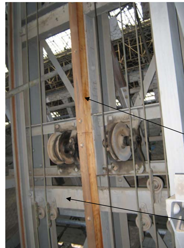
Figure 3-23: Wood Members at Elevator
