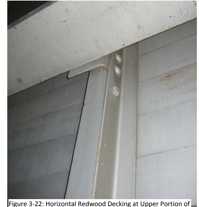
Figure 3-22: Horizontal Redwood Decking at Upper Portion of Hangar
