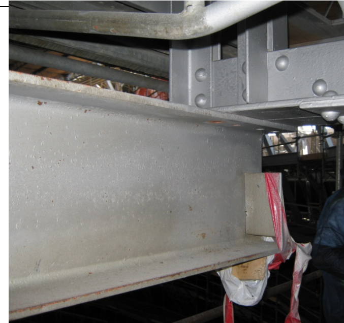
Figure 3-25: Crane Beam End Connection
