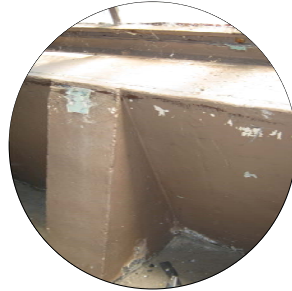
Figure 3-16: Concrete Wall at Hangar Perimeter, From Inside
