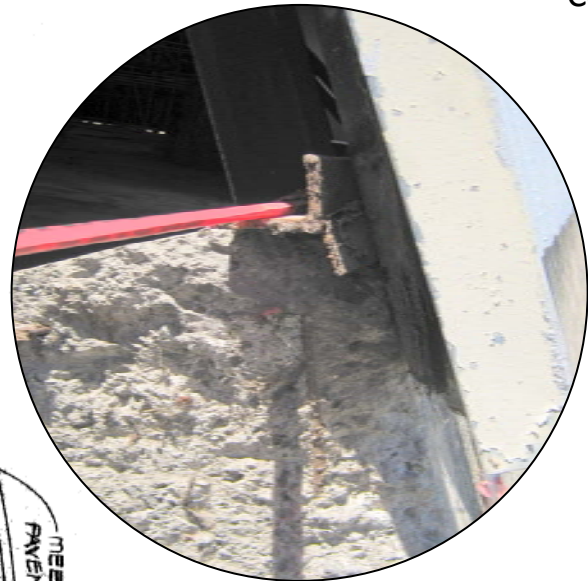
Figure 3-27: Saw Cut Concrete Wall at New Opening in Hangar
