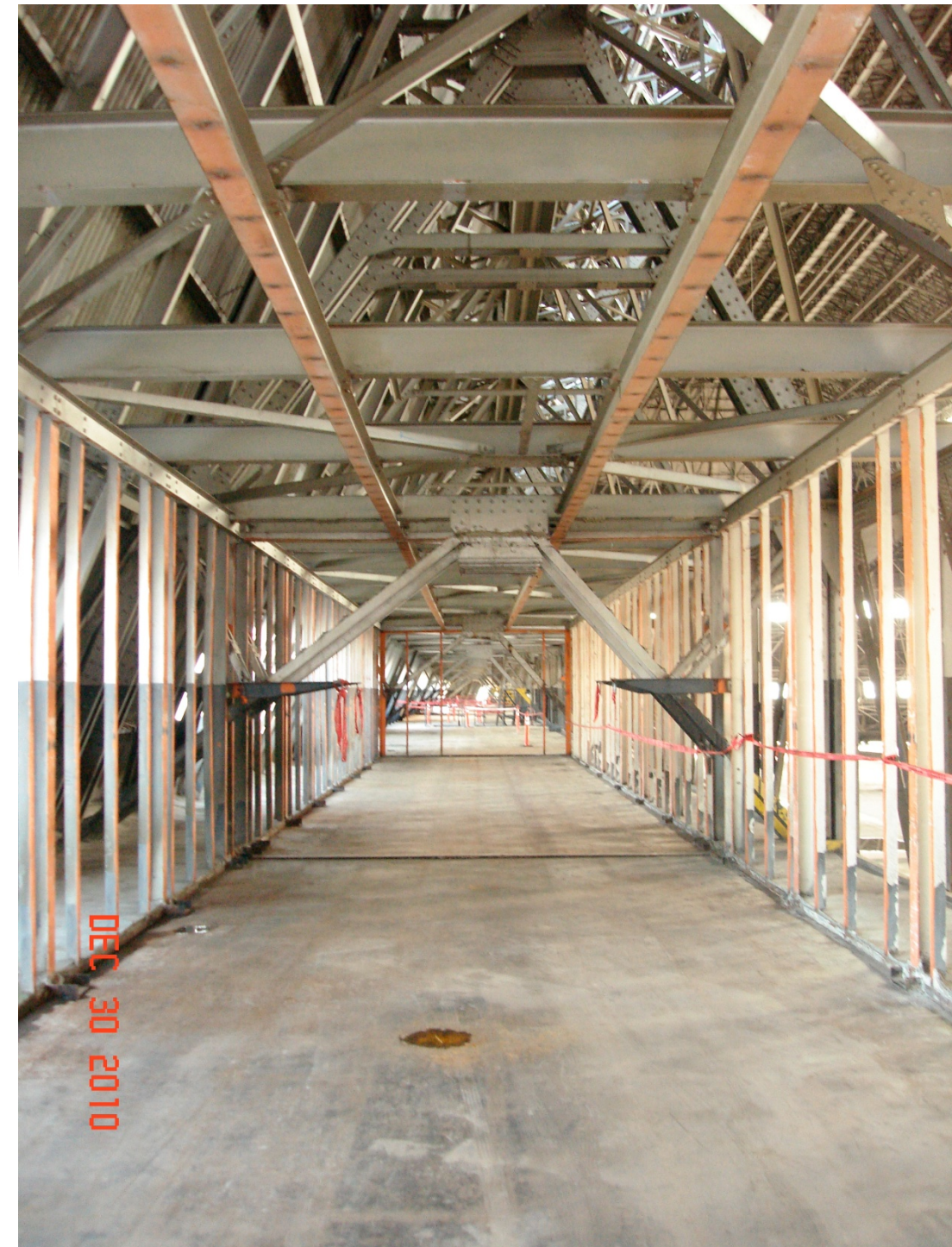
Figure 3-25: Interior Area of Cell Room at Mezzanine
