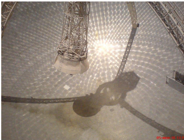
Figure V.A.3: View of 54m diameter spherical primary reflector of millimeter-wavelength radio telescope in Armenia. The on-axis corrector is seen mounted at the end of a pivot arm supported by a tripod structure.
