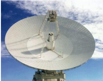
Figure 4. The 70-meter (230 feet) antenna at the Goldstone Deep Space Communications Complex in the Mojave Desert, California. This is one of many radio antennae at Goldstone, which is one of the three facilities that make up NASA’s Deep Space Network. (Image courtesy: NASA/JPL)
