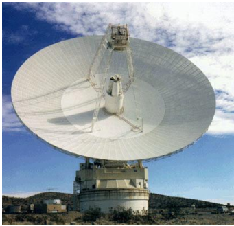
Figure 5. The 70-meter (230 feet) antenna at the Goldstone Deep Space Communications Complex in the Mojave Desert, California. This is one of many radio antennae at Goldstone, which is one of the three facilities that make up NASA’s Deep Space Network. (Image courtesy: NASA/JPL)
